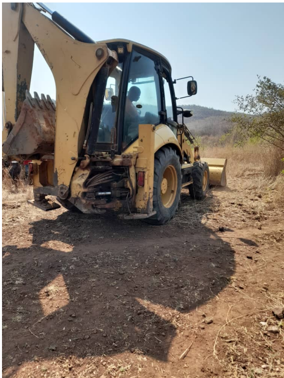
JCB onsite repairing hill top access roads
