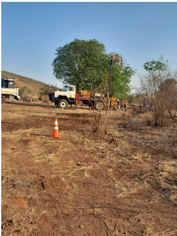
Drill rig and drill site
