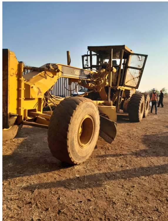
Grader on site maintaining access road
