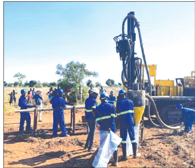
Air-core rig drilling its first hole at Kasiya
