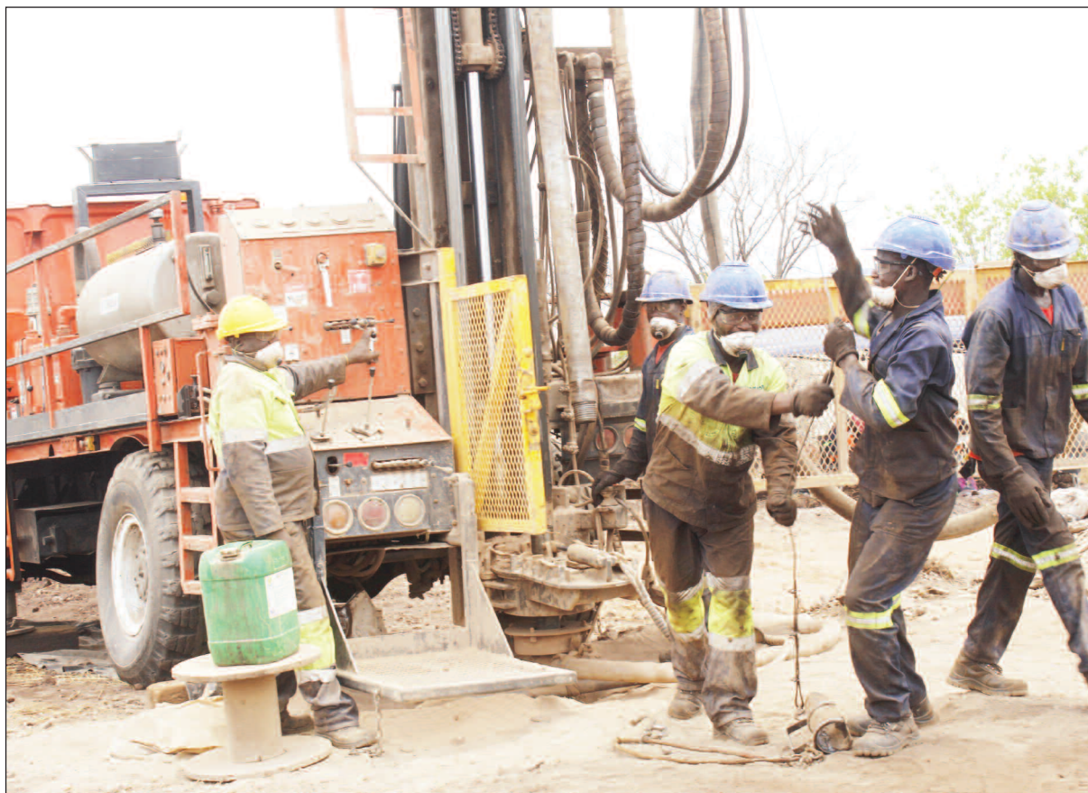
Drilling work at Kangankunde hill
