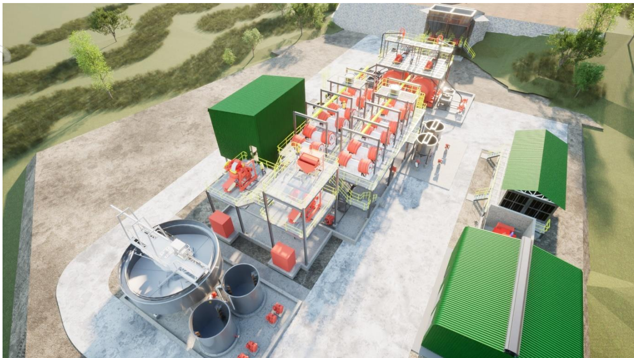
Image 5: Elevated view of the recovery circuit and tailings thickener.
