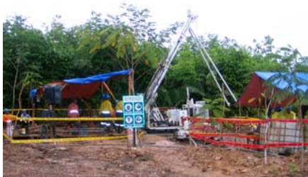
Diamond drill (PQ3) operations at Uyajan.
