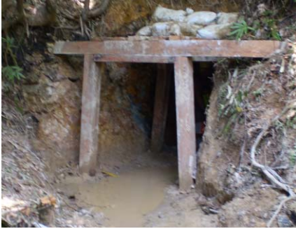
Exploration adit development.
